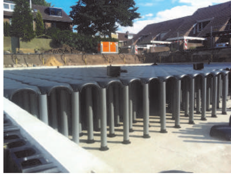
Installation between retaining walls
