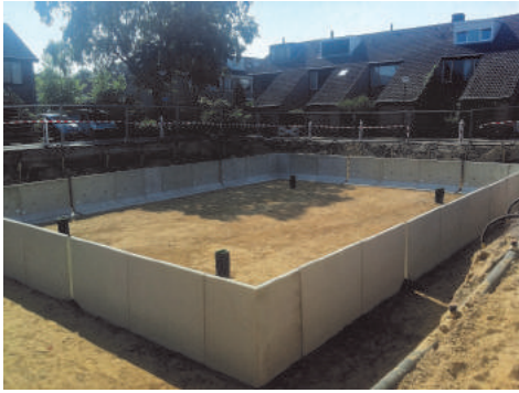
Use of durable drainage material
